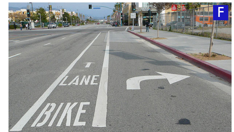
Example of a through bike lane.
