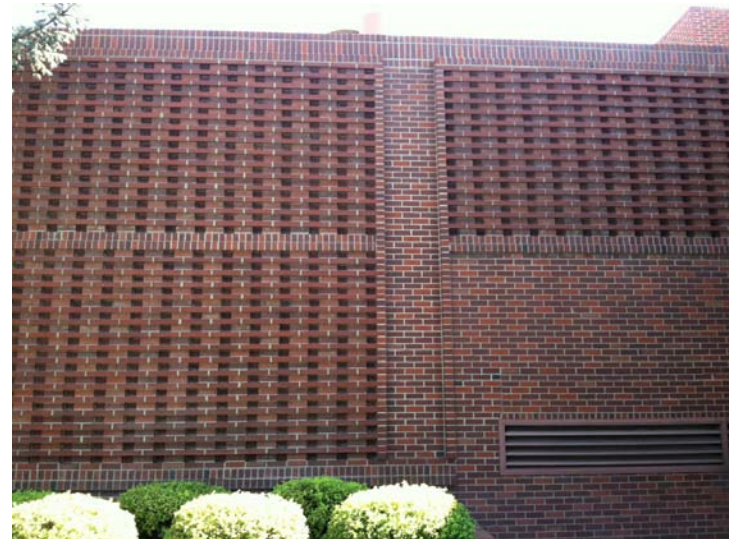
Brick used as a screen for mechanical equipment at St. Luke's Boise Medical Center creates an ornamental pattern on the building exterior.
