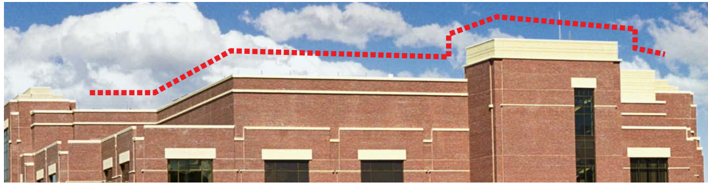
A building on the St. Luke's Boise campus that illustrates how St. Luke's uses a flat roof along with steps in the parapet.
