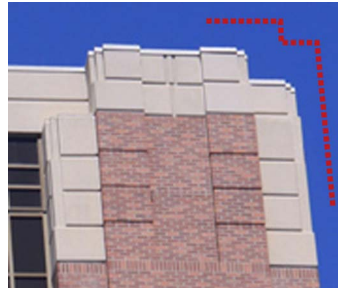
Corners of St. Luke's buildings are typically identified by steps in parapet heights as well as depth. This creates a strong element that represents the St. Luke's brand.
