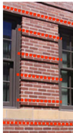
Banding in the brick aligns with adjacent building elements, tying together separate parts of the building.
