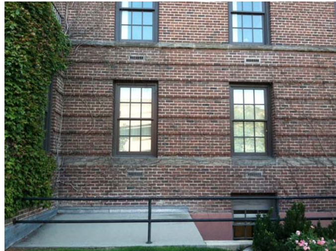
Use of reveals and coursing in the brick to create a base at the 1927 St. Luke's Boise hospital.
