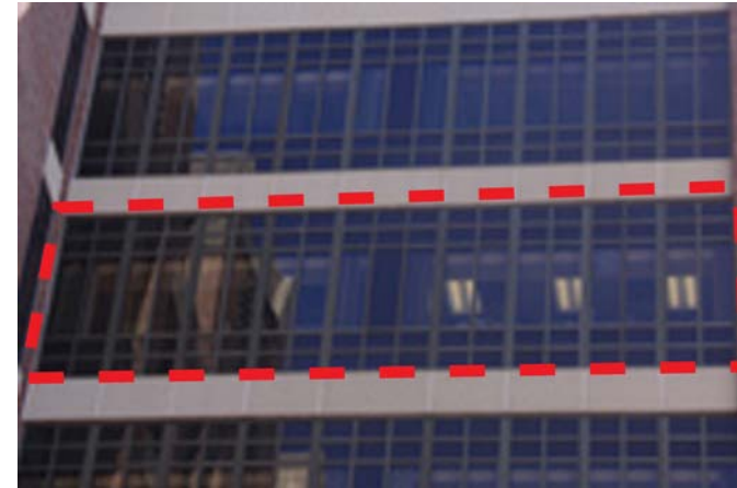
Glazing is broken up with mullion patterns and EIFS at St. Luke's Boise.
