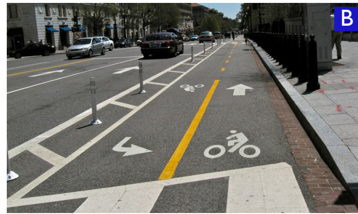
Example of a two-way cycle track.
