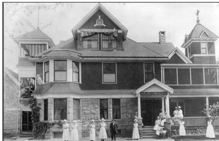
St. Luke's Hospital, 1903.
